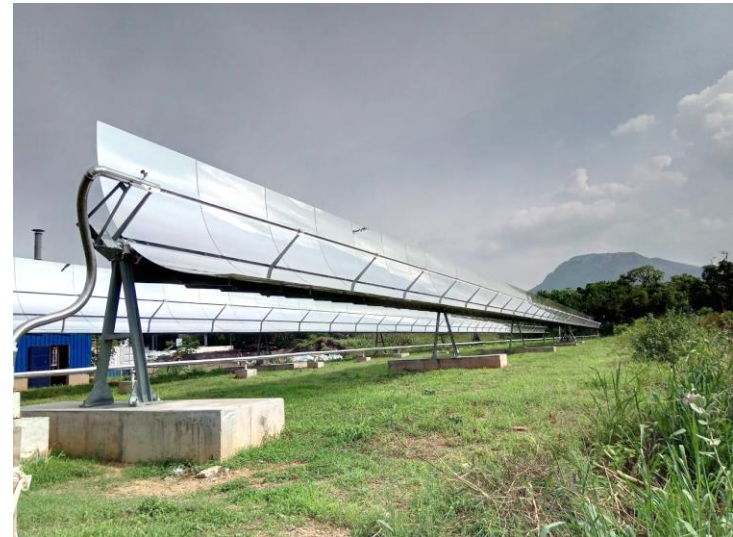
Solar CST system in Salem, Tamil Nadu
