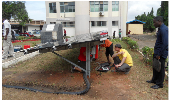
Installationsschulung an der Accra Polytechnic – Installation training at Accra Polytechnic
