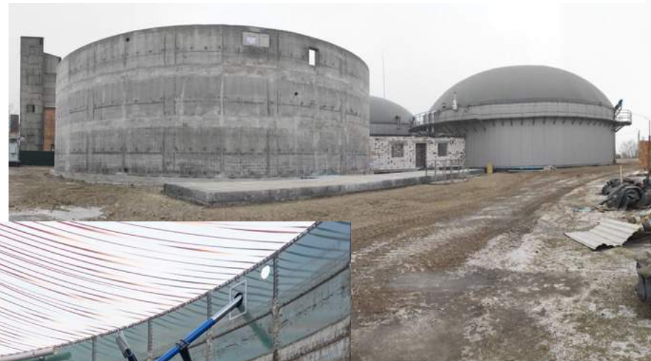
5,000 cbm digester for side entry mixer
