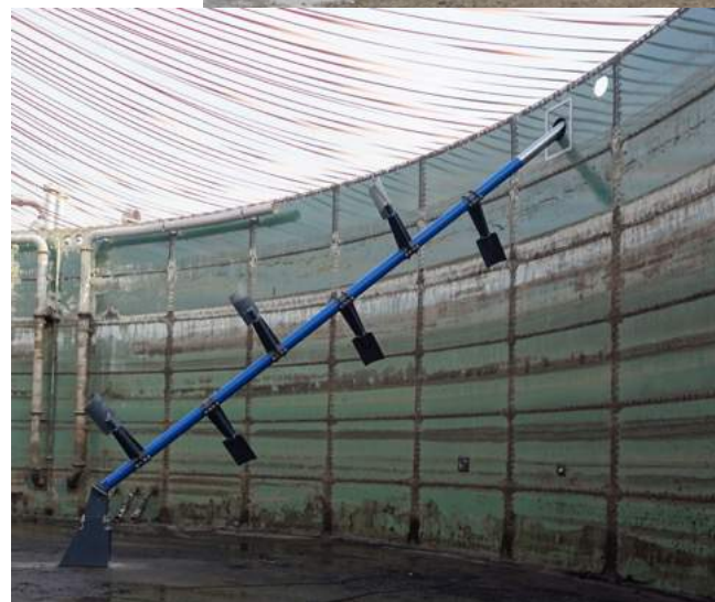
Optimization of a steel CSTR (7,000 cbm) with side entry mixers
