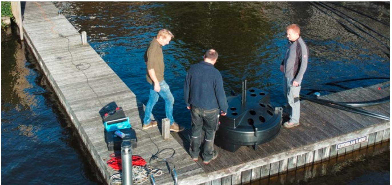
Installation of the FRANK WET surface water-source heat exchanger using a sturdy protective housing attached to the outer shell of the system with stainless steel cables
