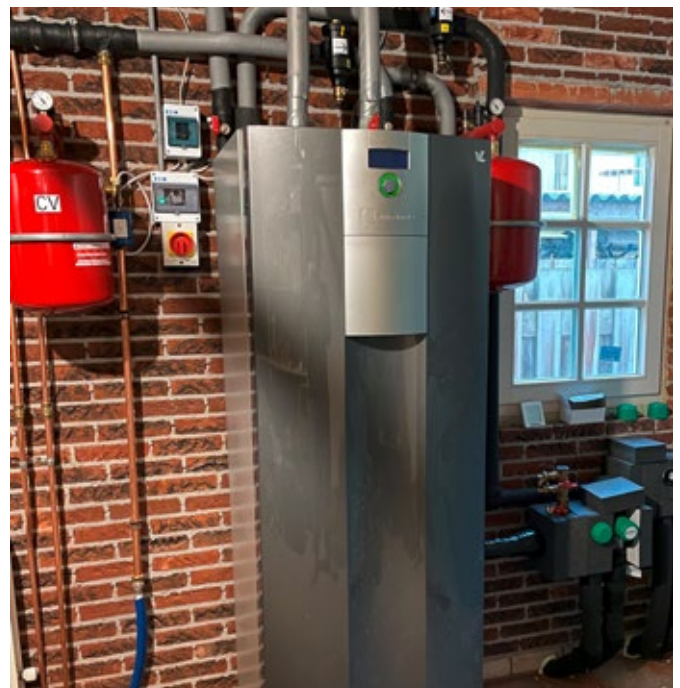
Heat pump for heating and cooling the building and insulated modular type-3060 brine distributor from Frank GmbH
