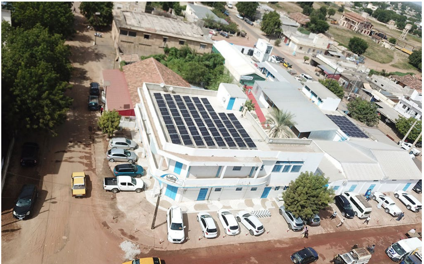
Over view Sidy Diop building with roof PV plant which supplies the KTI ice machine
