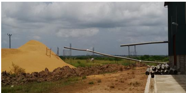
Figure 1: GADCO's site view – husk storage (left), production facilities (right), piping for transportation of husks.
