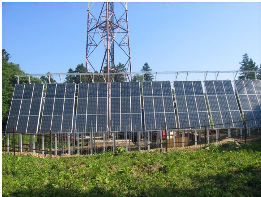
Figure 23 Autonomous 10.8 kW PV system, "MTS" mobile phone station for signal transmission, Lago-Naki, Krasnodar Krai
