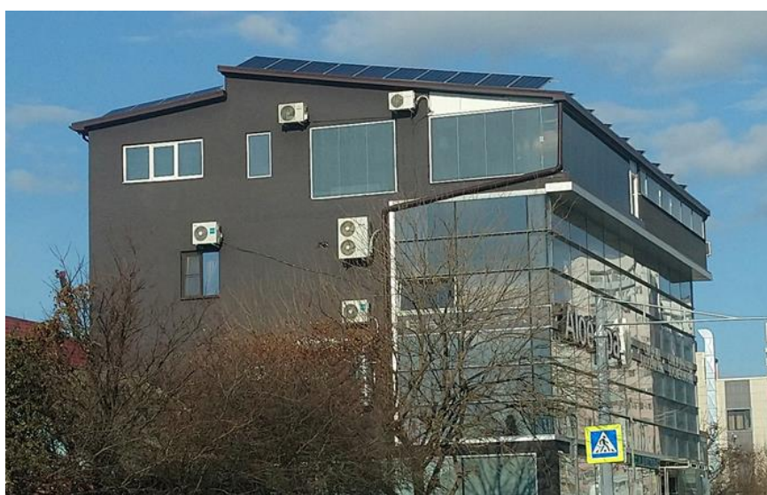
Figure 22 Hybrid PV-grid system; rooftop 30 kW PV solution on the roof of "Aloe Spa" Center in Krasnodar
