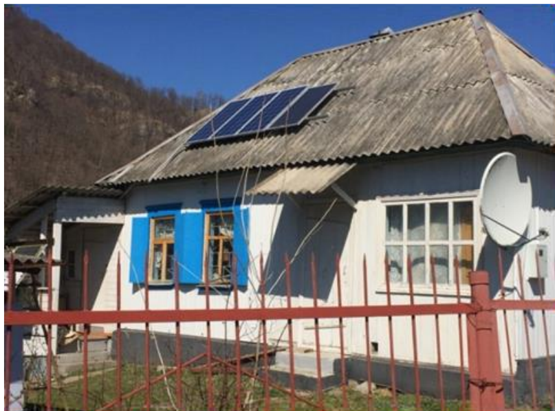
Figure 24 Autonomous rooftop PV system in Nikitino, an off-grid village in mountainous areas of Krasnodar Krai
