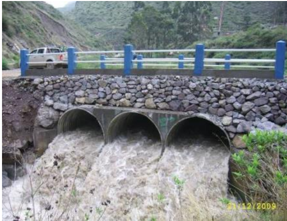
Construction of bridges
