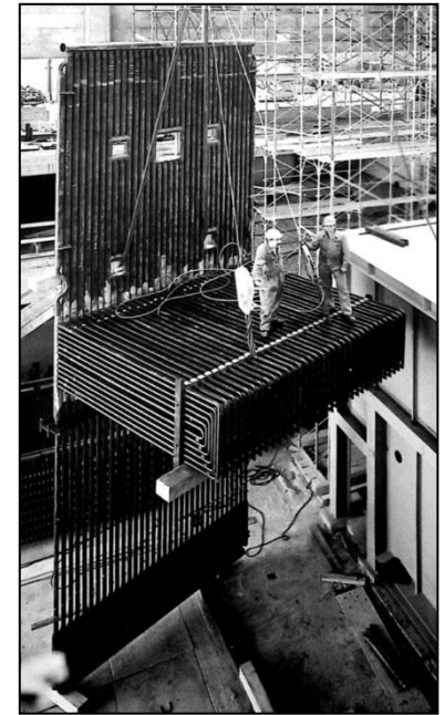
Evaporator flags - ERK invention (1958)
