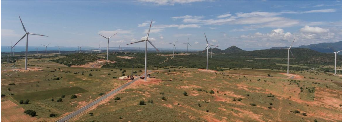
Phu Lac wind farm 24 MW, Binh Thuan province, FiT = 7.8 USct/kWh
