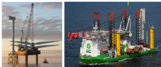
Turbine Installation (TIV)
