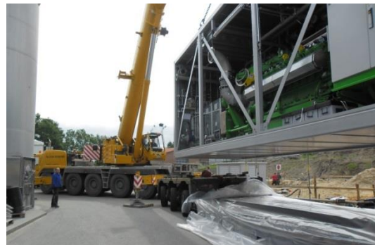
trucked to site
