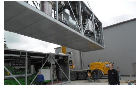
assembly on site
