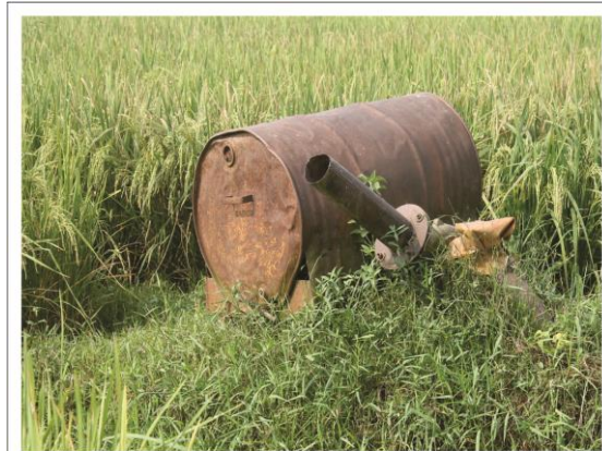
Traditional Diesel Pump
