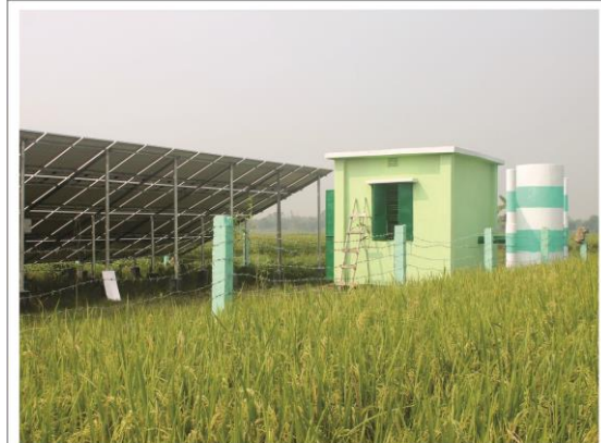
Solar Irrigation Pump
