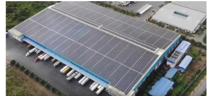
Mekong Logistics, Vietnam 2.42 MWp
