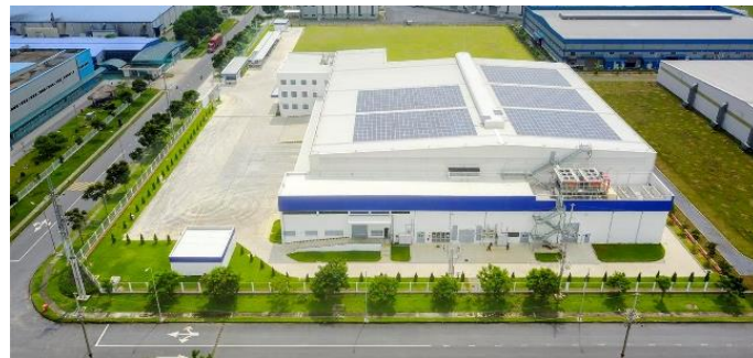
Emergent Cold, Vietnam 308 kWp
