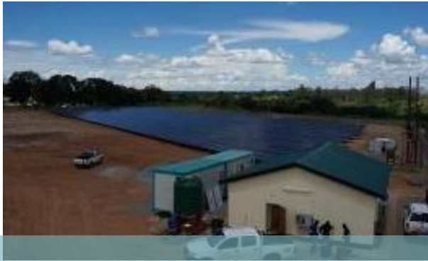
Copperbelt Energy Corporation Sambia, 1 MWp
