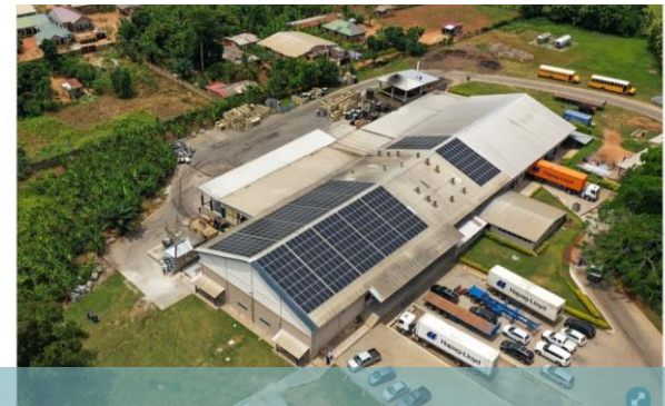
Bomarts Farms Ghana, 173 kWp
