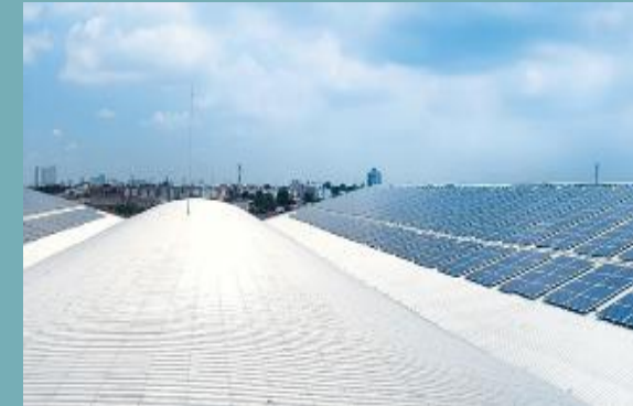
Star Aire, Thailand 1 MWp
