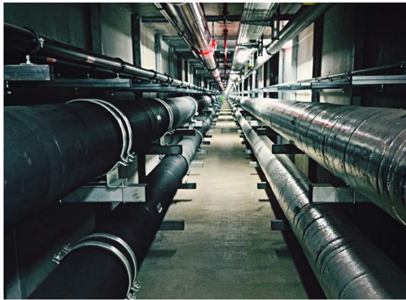
Figure 24: District heating tunnel
