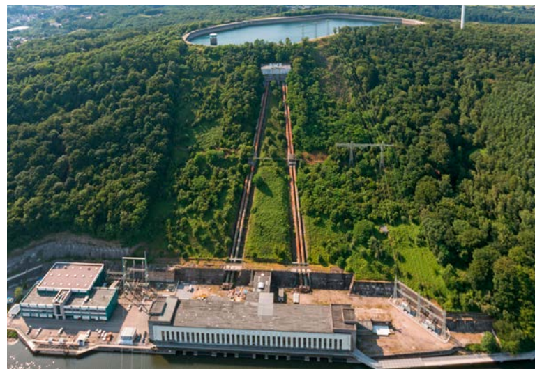
Figure 21: View of the pipes on the power house of a pumped storage station
